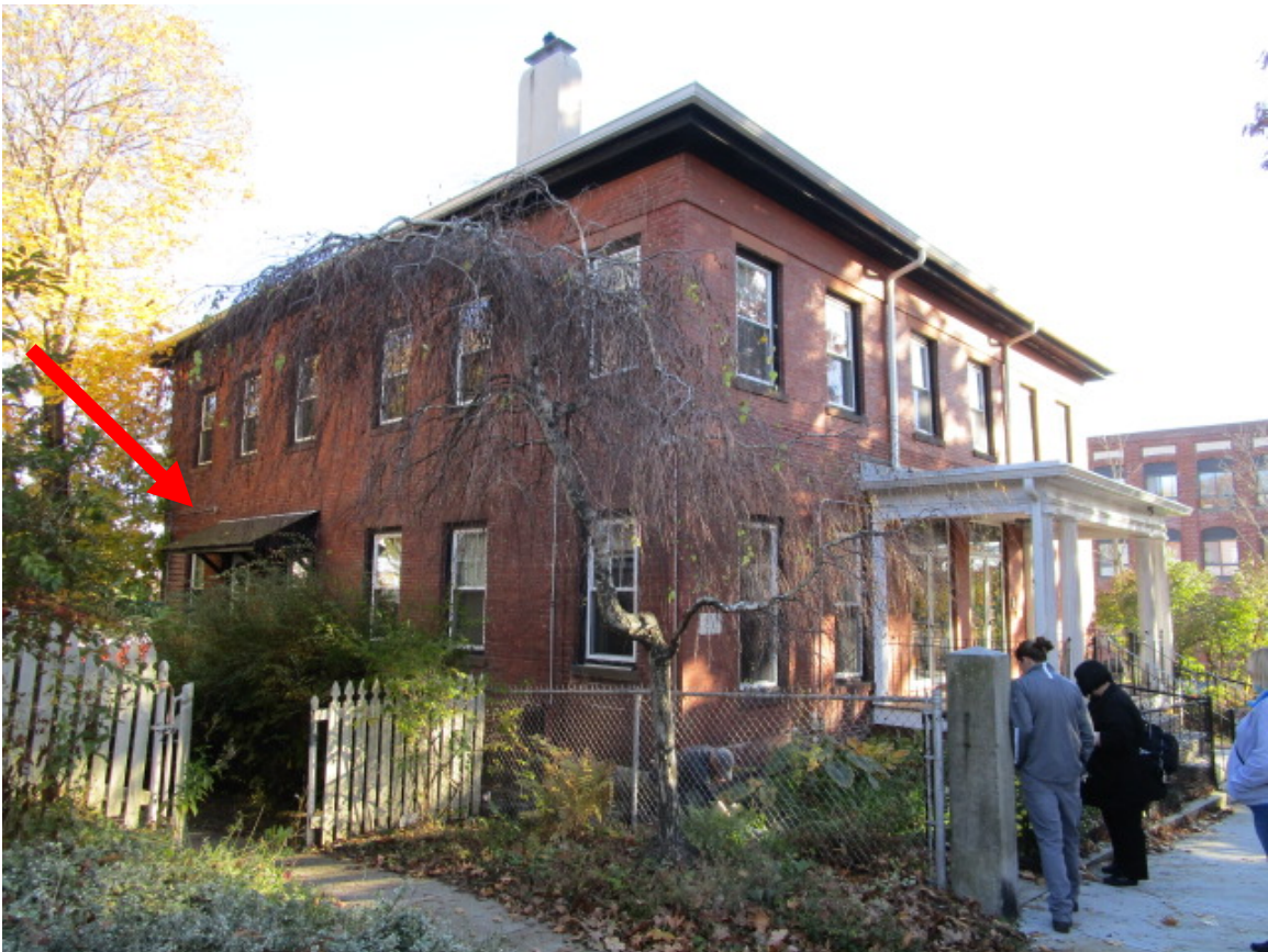
2. 21 Crown Street façade and north elevation
