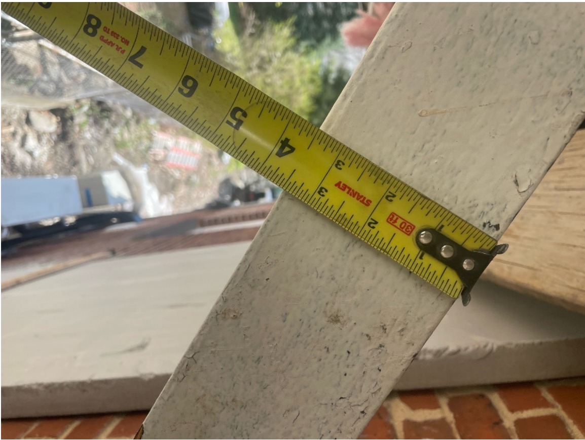
5. 21 Crown Street north elevation entrance, note use of modern lumber
