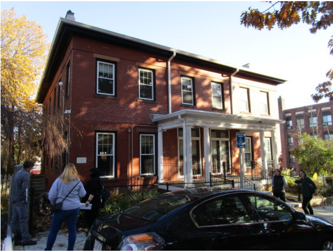
1. 21 Crown Street façade and north elevation
